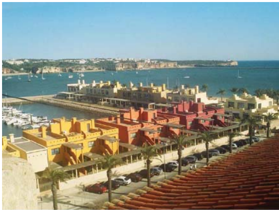
Photo 1 - The vulnerability of these buildings is very high.
